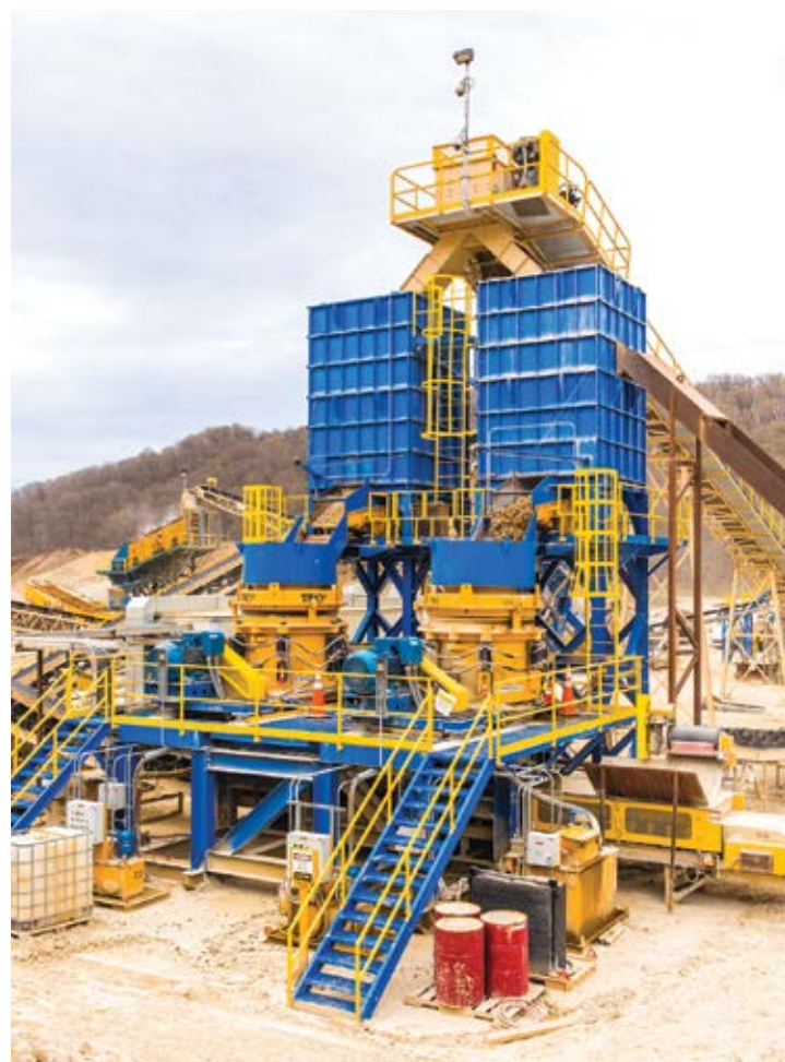
Trio crushers in an aggregate application. (Photo: Weir Minerals)
