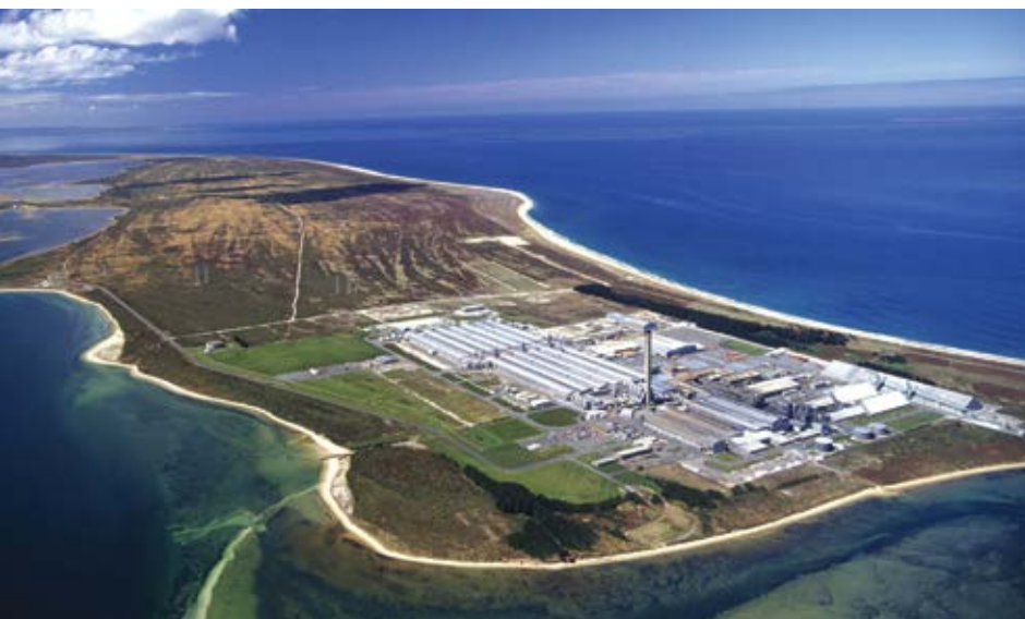
A new electricity agreement extends the life of the Tiwai Point smelter (above) until the end of 2024.
