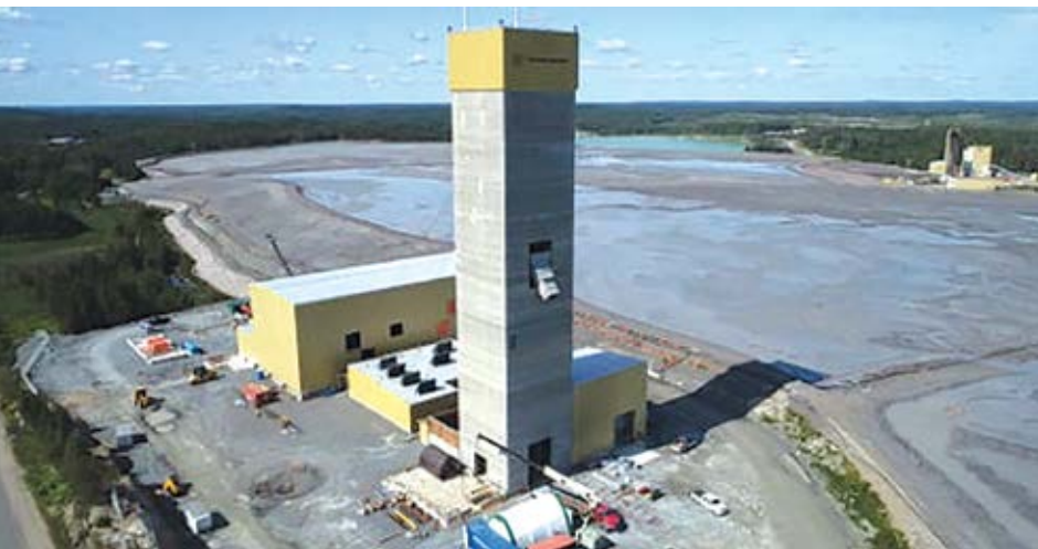
The Macassa No. 4 shaft project (above) is advancing ahead of schedule.
