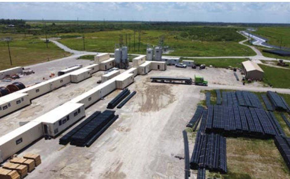
Tubi USA modular plants manufacture HDPE pipe on-site. (Photo: Tubi USA Inc.)
