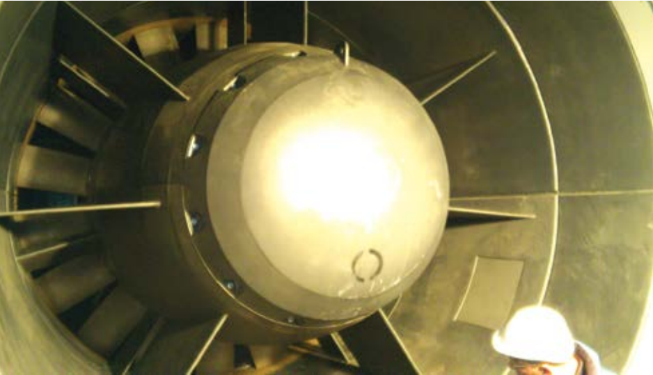
Above, the nose fairing of the axial fan system offered by CFE Technology GmbH. The system offers fully automatic operation, a smaller overall footprint, and significantly improved airflow control over competing centrifugal fan-based solutions. (Photo: CFE)
