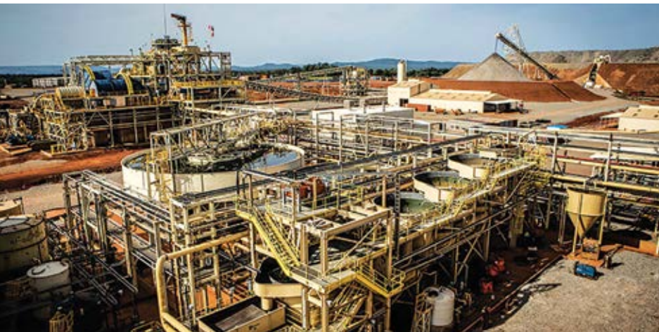
B2Gold successfully increases Fekola's mill capacity to 7.5 million mt/y.
