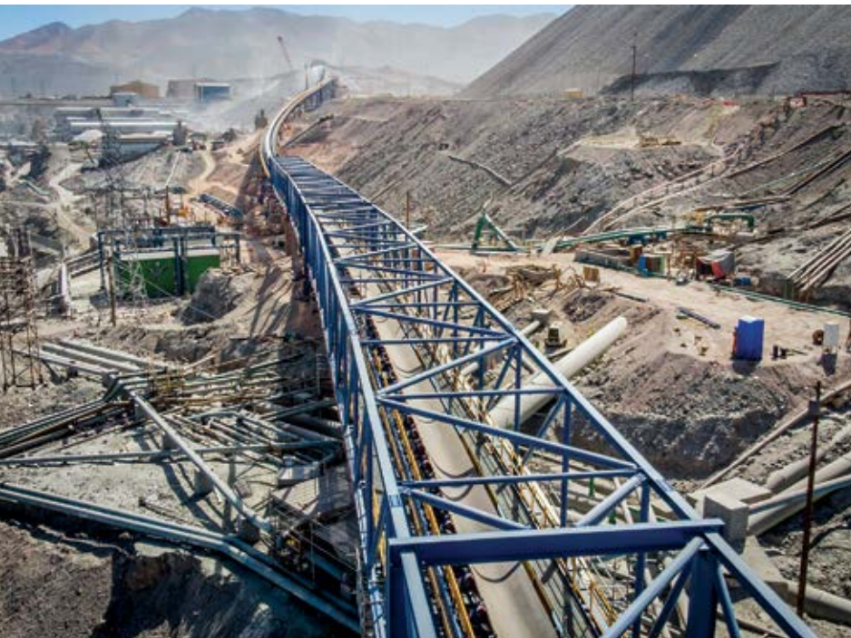
The overland conveyor passes over infrastructure that has accumulated over 100 years.
