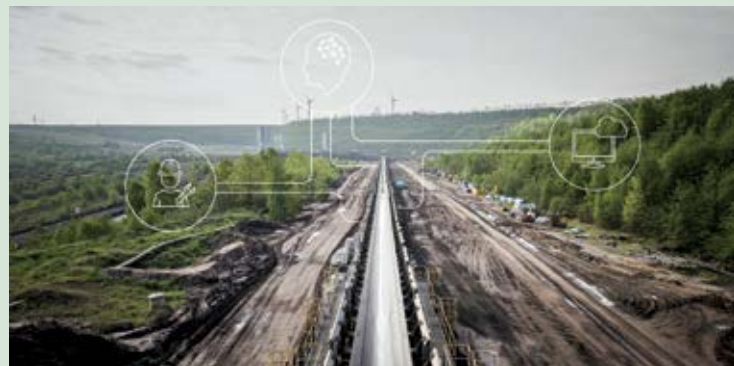
BeltGenius ERIC (Efficiency and Reliability Intelligent Control) from Voith is a software solution that analyzes a range of data to determine how efficiently the belt conveyor systems of a mine are operating.
