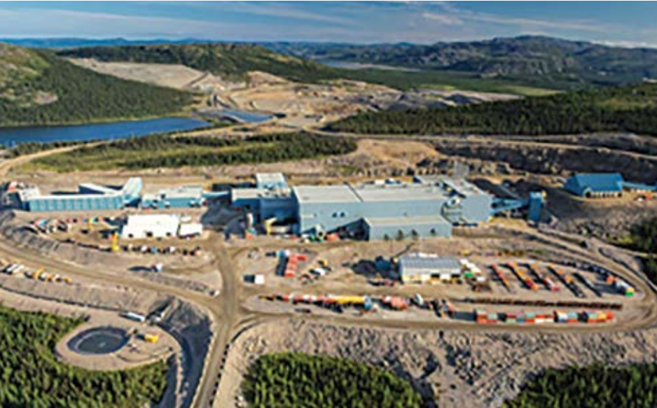
A fly-in, fly-out operation, the Voisey's Bay mill (above) processes 6,000 metric tons per day. (Photo: Vale)
