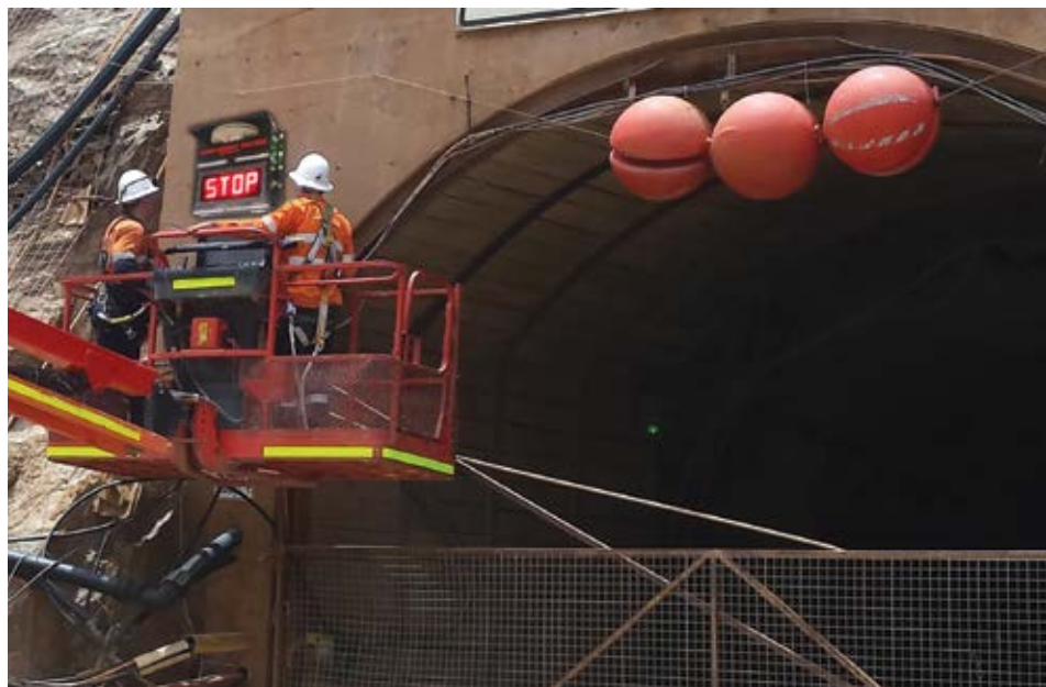
This laser-based warning system developed by RCT warns drivers that the equipment they're operating may be too tall to enter the mine portal, a common problem encountered when drivers forget to lower the truck body on re-entry.
