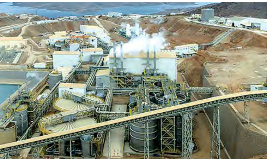
Alacer's pressure oxidation circuit (above) processes Çöpler's sulphide ore. (Photo: Alacer Gold)
