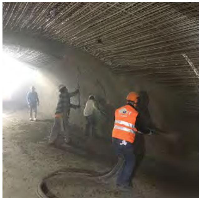
MAPEI's UTT products have commercial as well as industrial applications. Its additive technology was added to shotcrete to create the walls of this high-tech wine cave.
