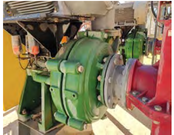
The Schurco slurry pump shown here feeds a cyclone, an application that requires precise and reliable pump performance.
