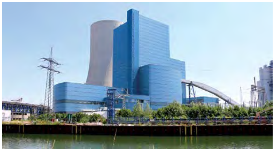
A new coal-fired power plant, Datteln 4 (above), is recently brought online in Germany.
