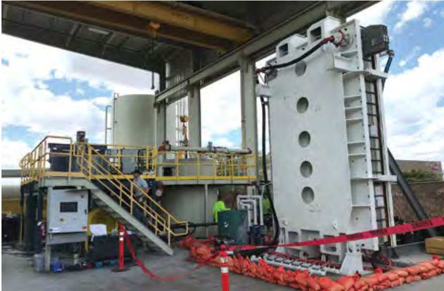
The 5 x 3 pilot plant that FLSmidth demonstrated in Nevada in late 2019.
