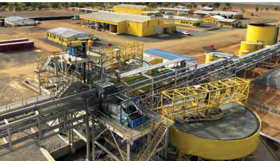
Endeavour will add two SEMAFO operations: Mana and Boungou. The Boungou carbon-in-pulp plant (above) has a 4,000-mt/d capacity.
