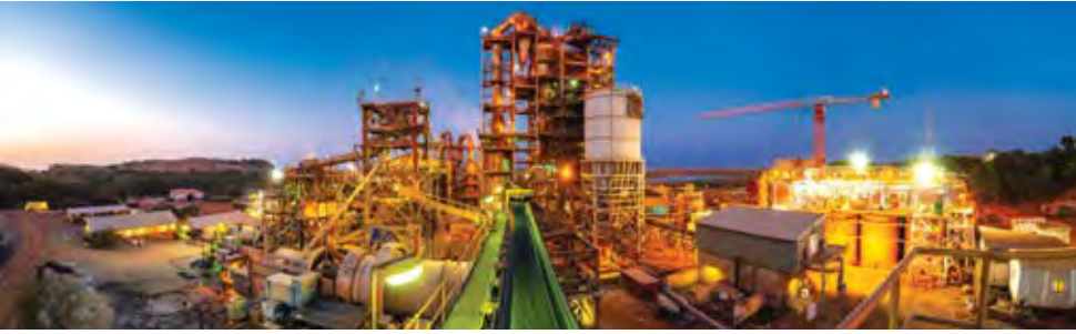
The roaster at the Syama perrocessing plant (above) was taken offline in early October due to the detection of a crack in the main external shell. (Photo: Resolute)
