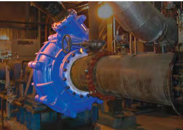
A Warman froth pump from Weir Minerals. Pumps are often overlooked in flotation circuit optimization but they are crucial to a smooth running operation. (Image: Weir Minerals)
